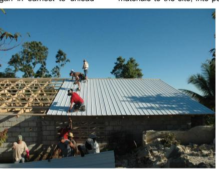
Putting the metal roofing over the new rafters.
