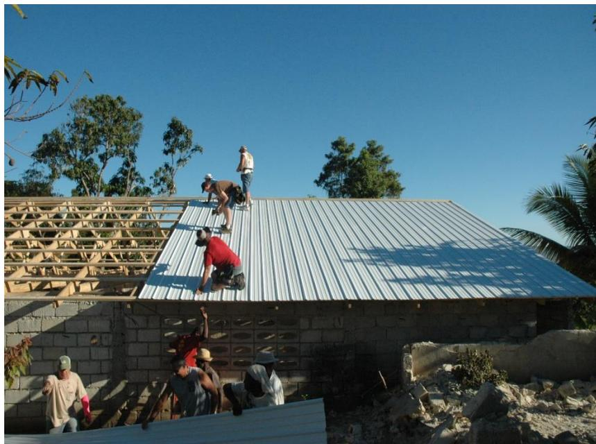
Putting the metal roofing over the new rafters.
